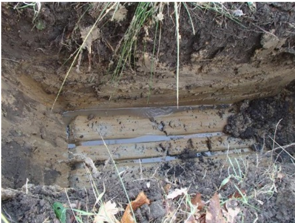
Photograph 8: TP1 GL to 1.0m begl
