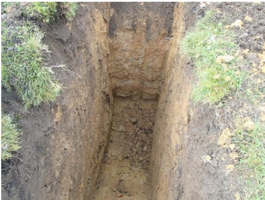
Photograph 16: TP5 GL to 2.20m begl
