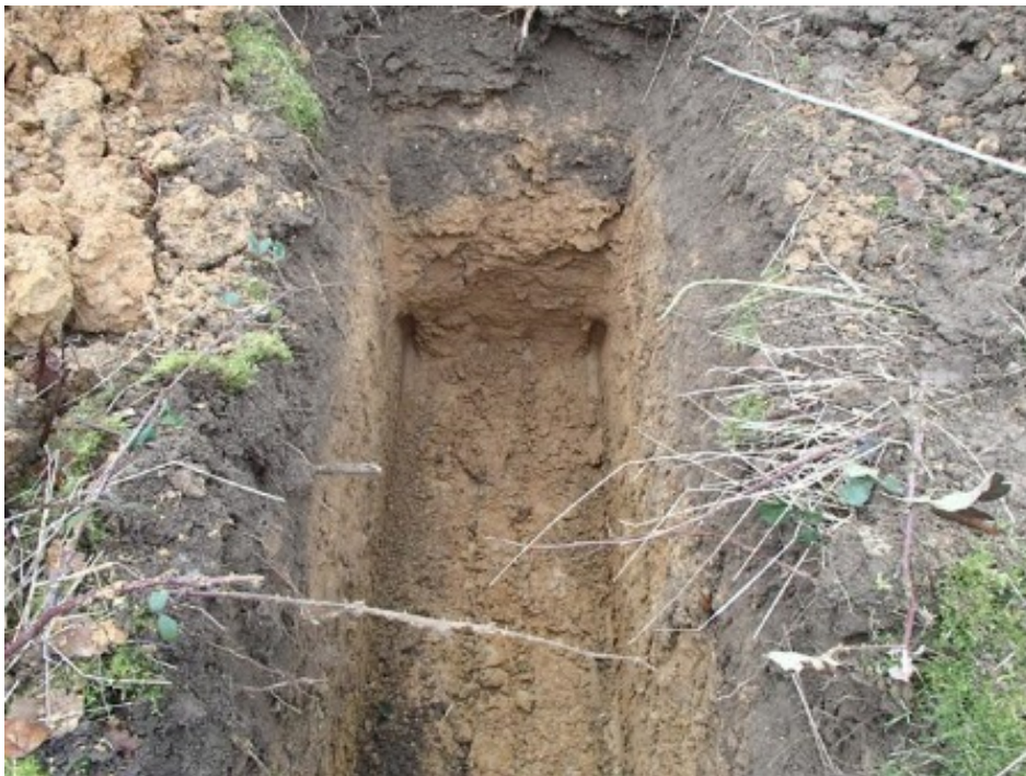
Photograph 10: TP2 GL to 1.20m begl
