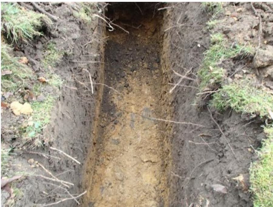
Photograph 14: TP4 GL to 1.30m begl
