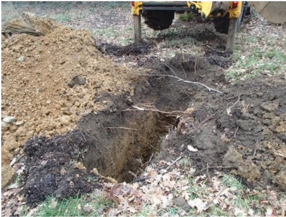
Photograph 17: TP6 GL to 1.80m begl
