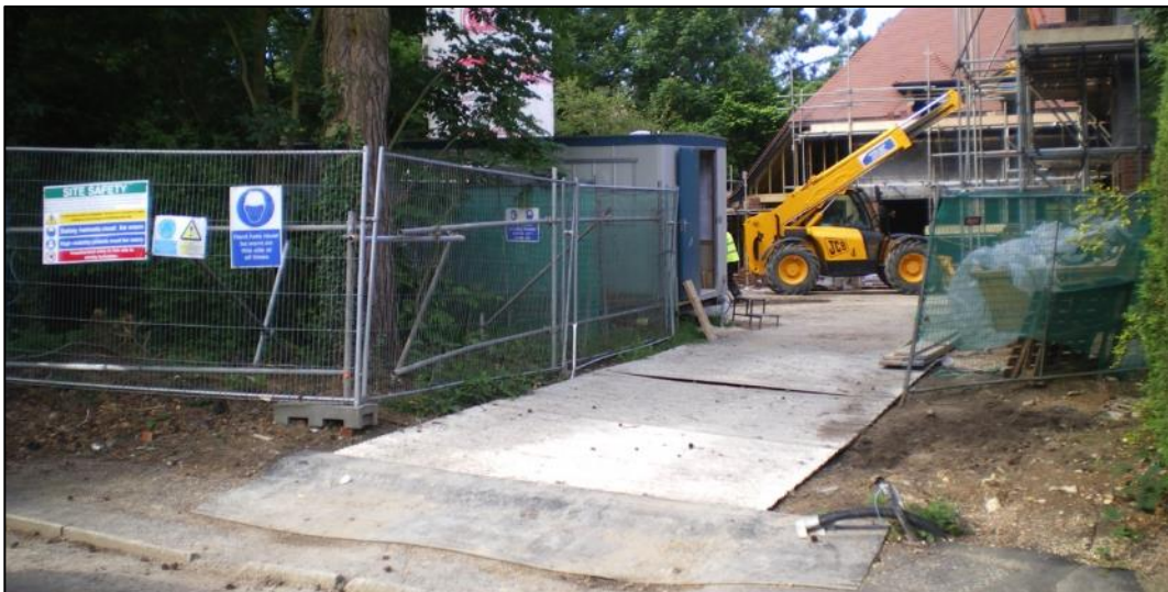
Vehicular ground protection trackway
