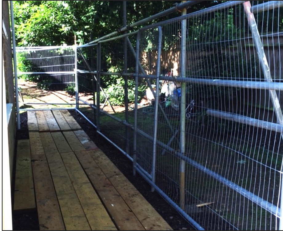
Scaffold board pedestrian ground protection
