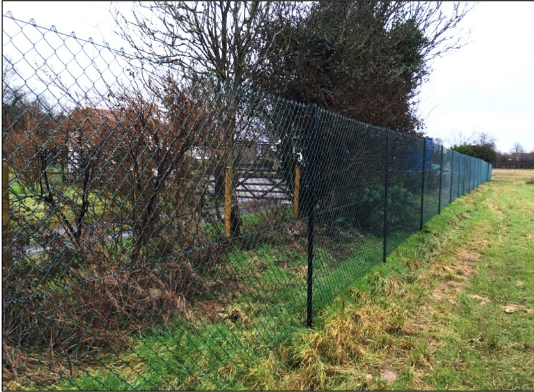
Chain-link on angle-iron uprights
