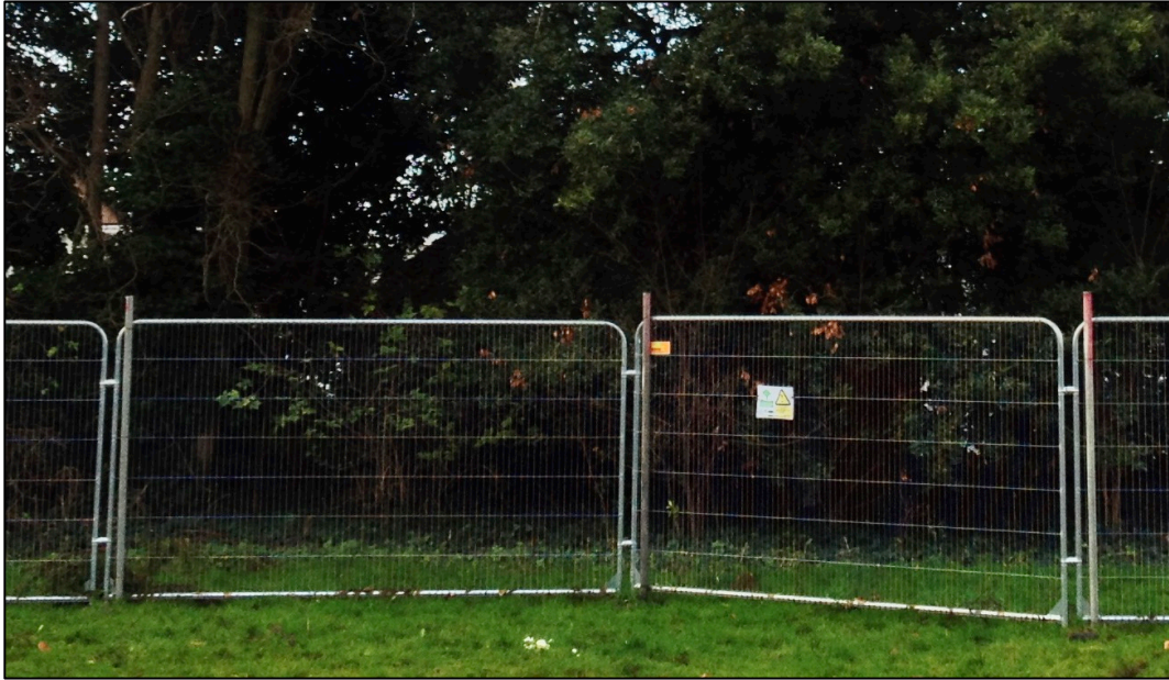
Weld-mesh panels on scaffold uprights
