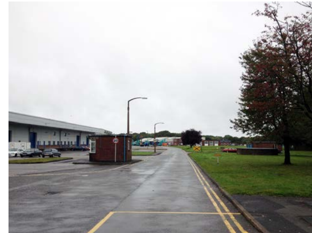
View into Chalcroft Business Park from outside the existing security lodge
