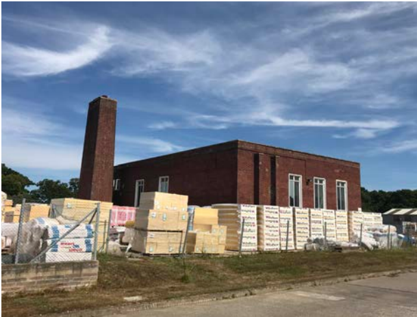
Unit 10 (to be demolished)
