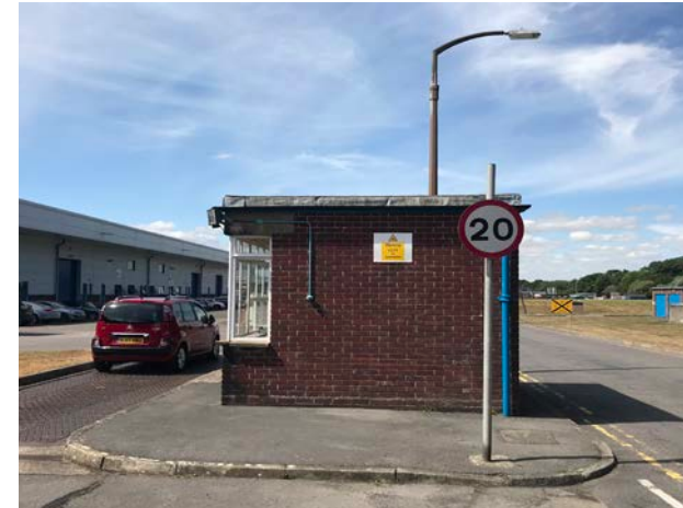
Weighbridge (to be retained)
