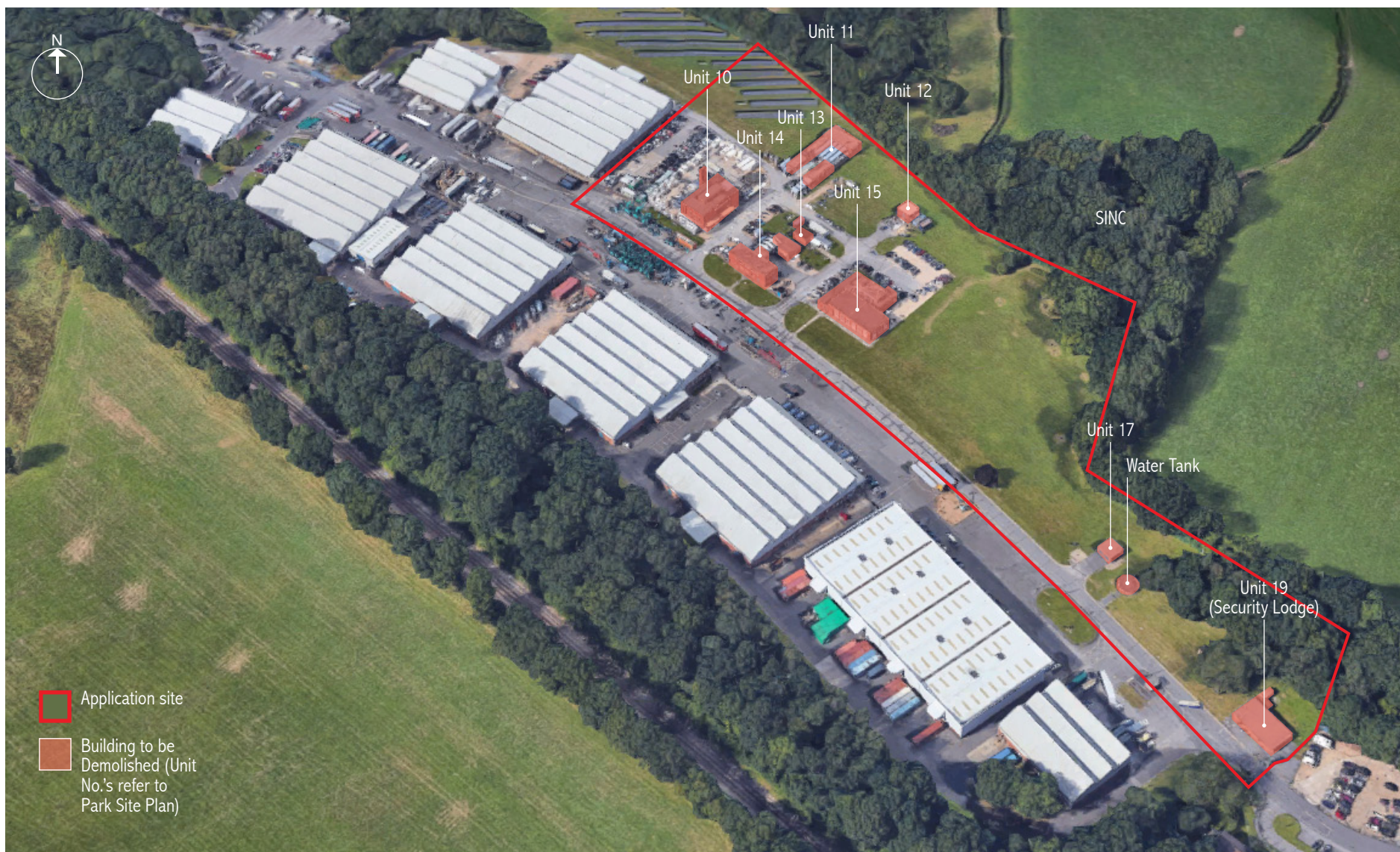
Proposed buildings to be demolished on site
