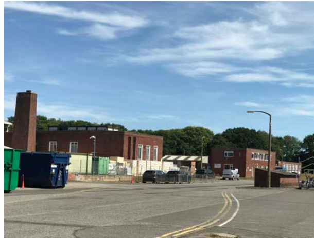
Estate access road looking east
