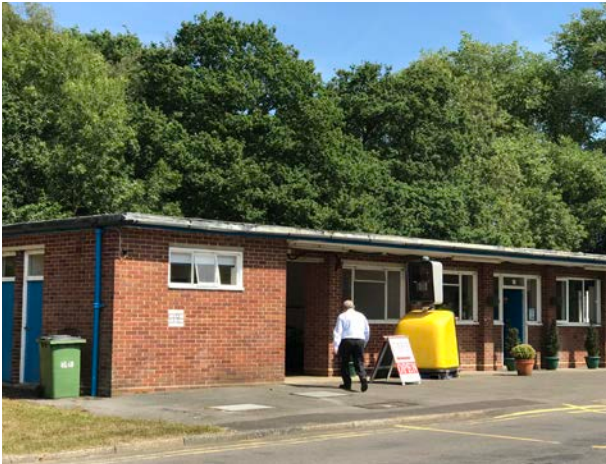
Security lodge to the Park (to be demolished)
