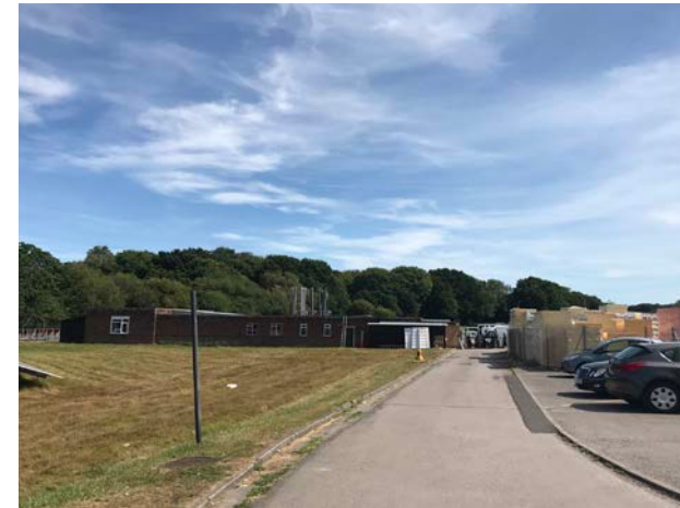
Unit 11 (to be demolished) looking east
