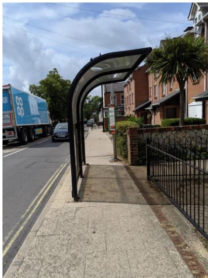
Photograph 4: Bus shelter on Station Road north east bound
