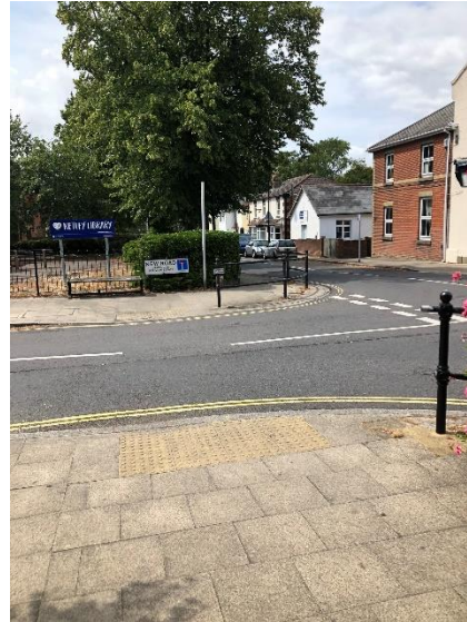
Photograph 3: Tactile pavement crossing on New Road
