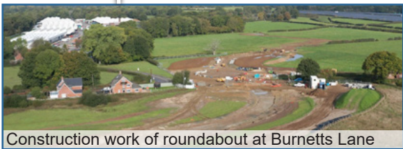
Construction work of roundabout at Burnetts Lane
