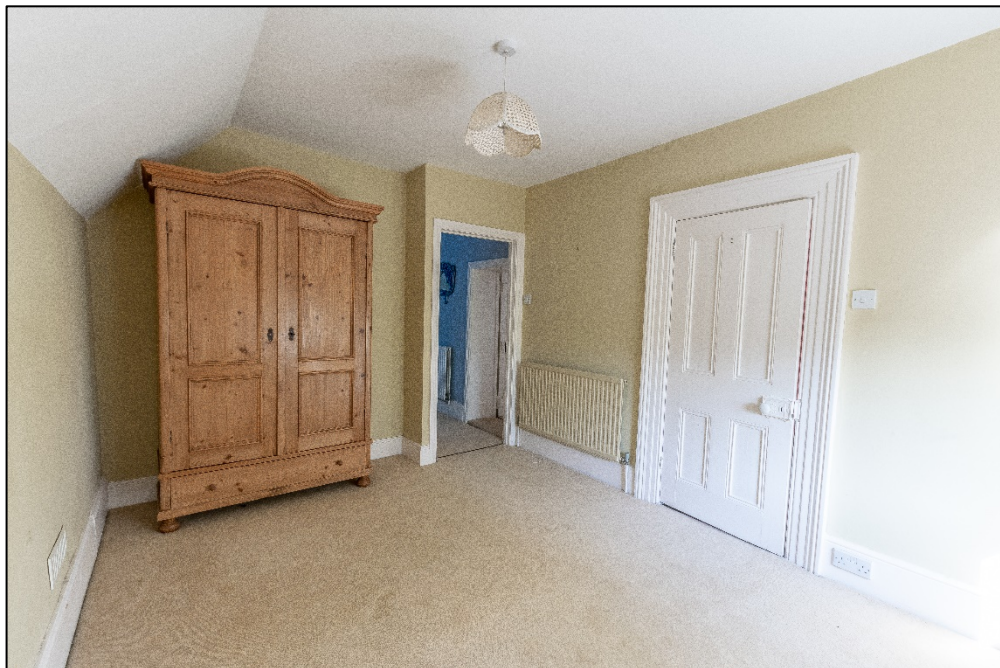
Photograph 27 Western-most bay in the south wing at first floor (Courtesy of EBC)
