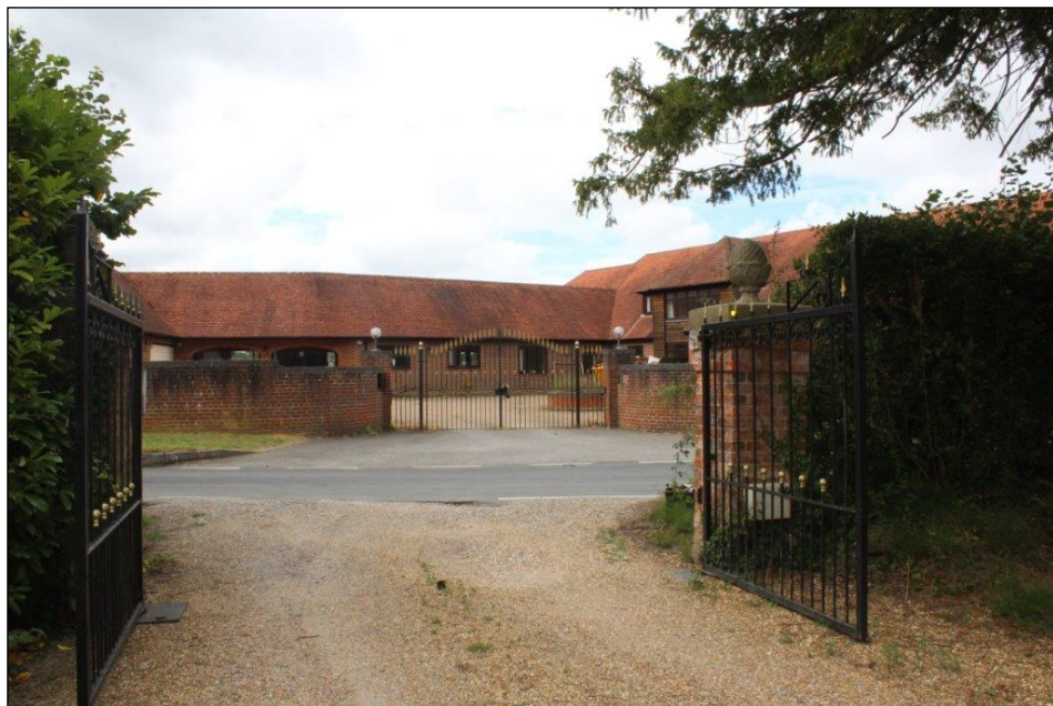
Photograph 38 Victoria House from the entrance drive to Firtree Lane
