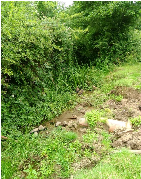
Plate 8: Reach 6. Southern channel poaching and scrub
