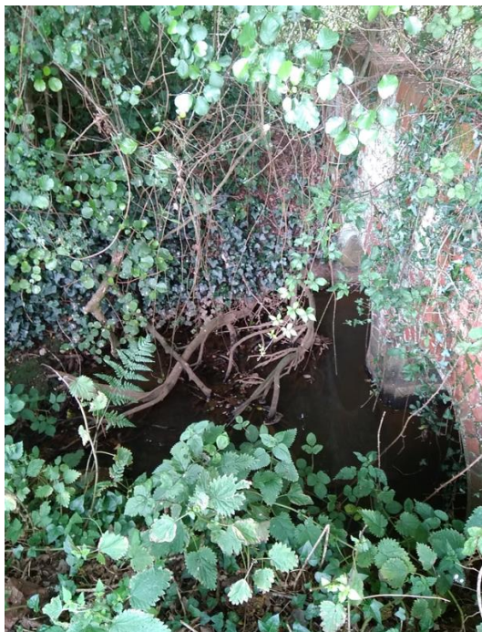
Plate 4: Reach 6. Inflow of southern boundary channel through twin culverts
