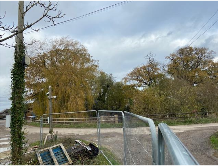
Plate 2: Security light on utility pole adjacent to a great crested newt breeding pond.
