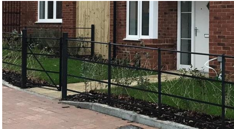
0.9m Estate railings
