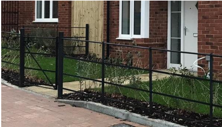
0.9m Estate railings
