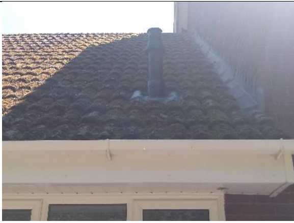
Photograph 5. Flue at north-east with raised tiles surrounding
