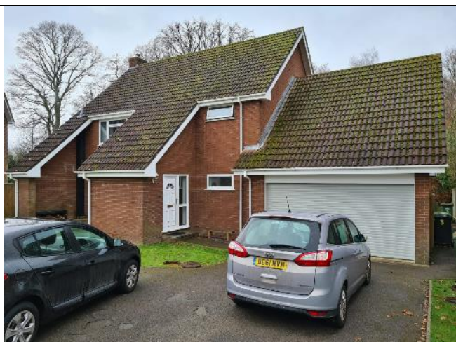
Photograph 3. Front elevation in a good state of repair
