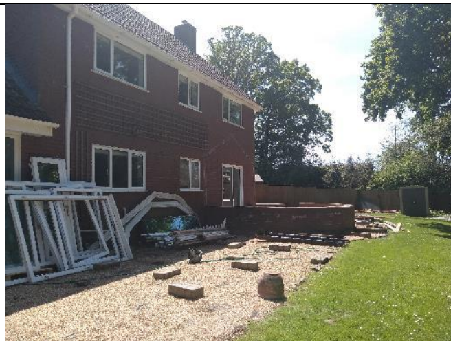
Photograph 2. Rear elevation hardstanding and amenity grassland
