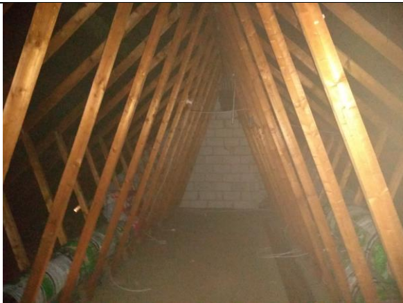
Photograph 7. Loft void facing west towards the location of bat droppings on the far wall
