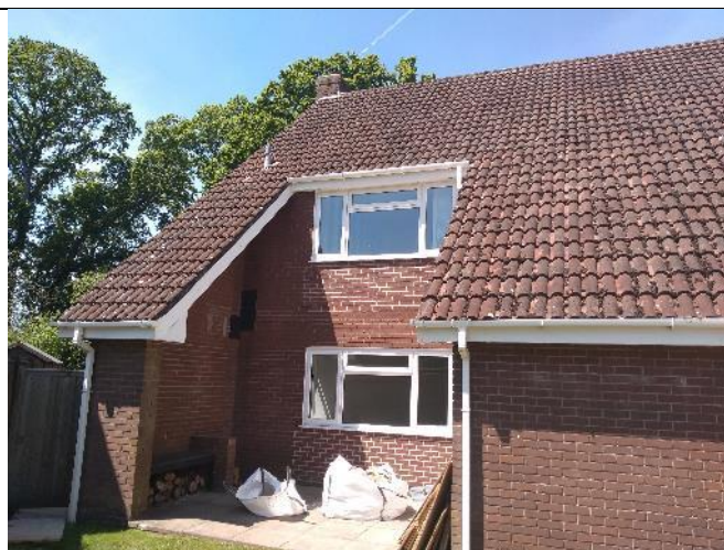
Photograph 4. South-west roof, flue with raised tiles surrounding
