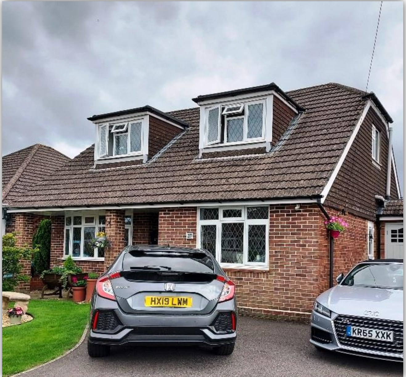
Dormer windows above the front elevation, side (west) elevation and hanging tiles.
