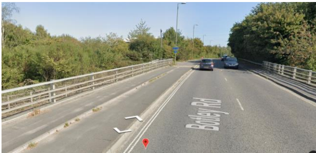
4. Site access off Botley Road viewed from M27 bridge. Adjoining footpath and cyclepath (Source Google StreetView)
