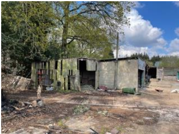
20. Barns, existing hardstanding and established screening along site boundary and to the west.
