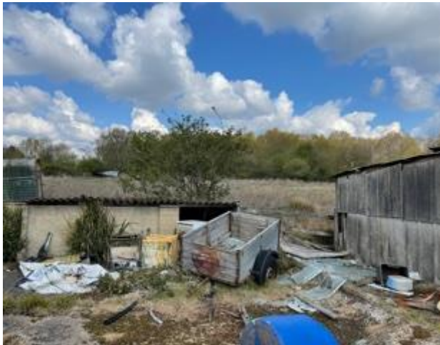
27. Barns and existing hardstanding. open land and established screening beyond to the north-west.
