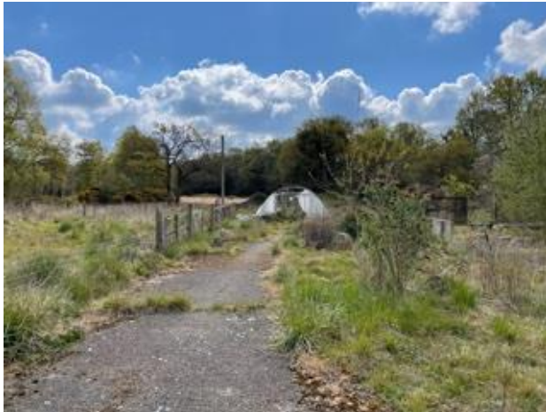
29. Existing hardstanding track leading to greenhouse
