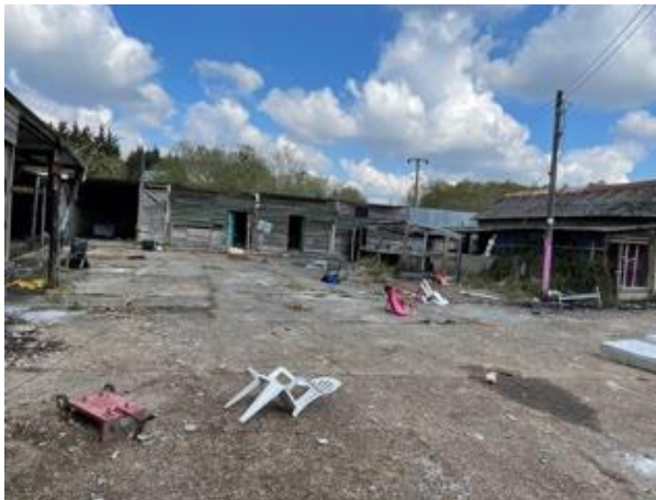
21. Barns and existing hardstanding. Established screening to the west.
