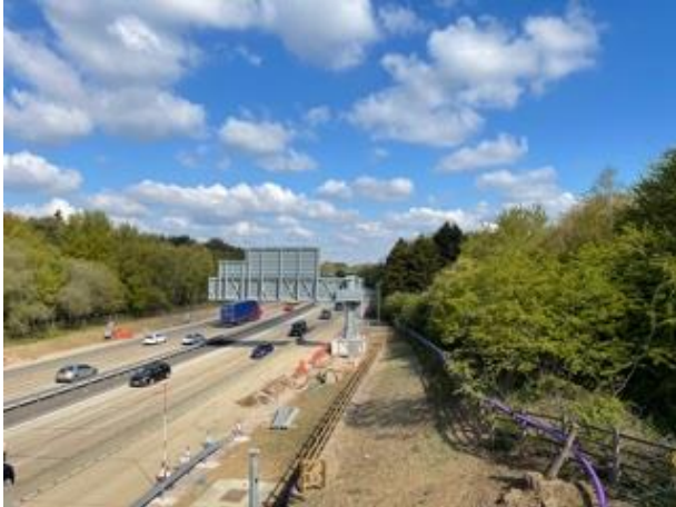
1. Long view of screened boundary to site access road and main site
