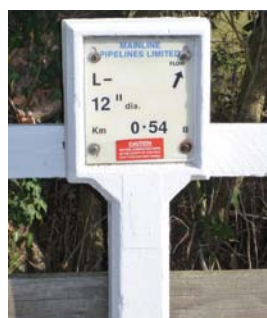
Mainline marker post
