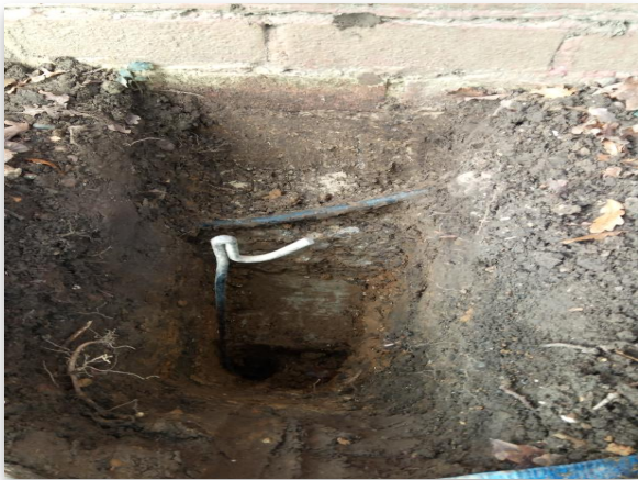
Fig 1.2: Trial Hole 1 Footing
