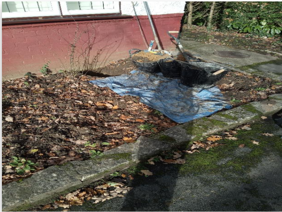
Fig 1.1: Trial Hole 1 Location
