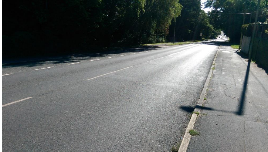
Photograph 1: Providence Hill (A27) Existing Conditions
