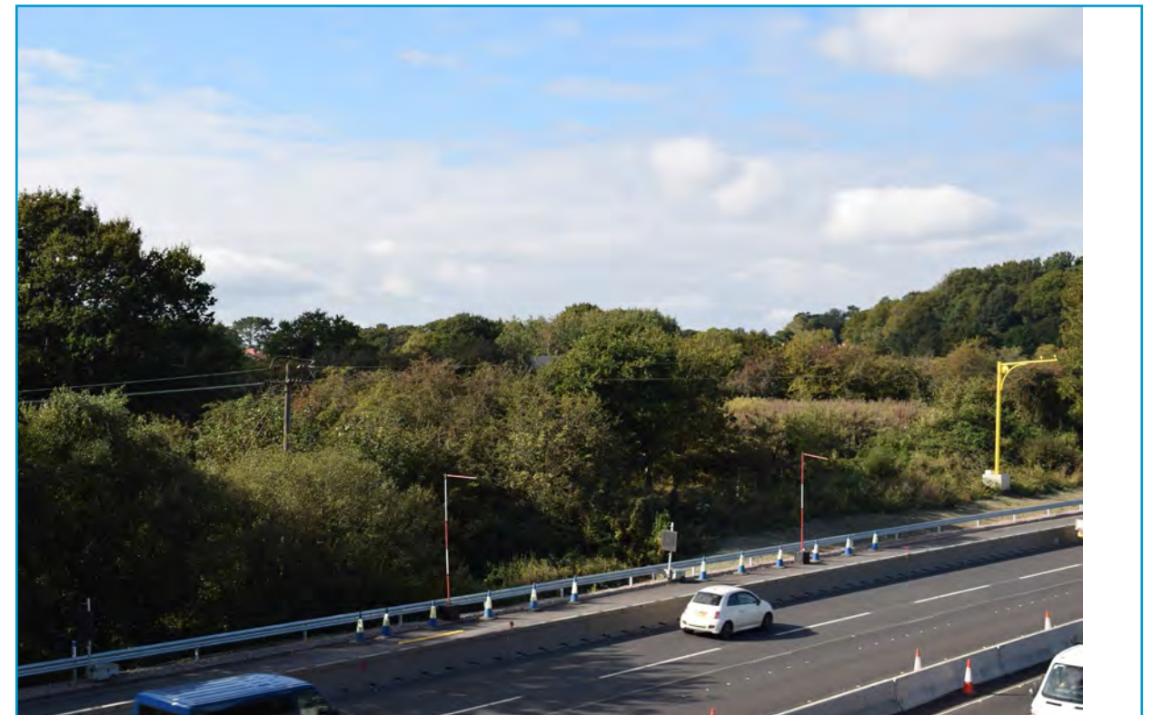
VP 15: Looking west from bridge over M27 on Dodwell Lane. No view of site due to intervening vegetation.
