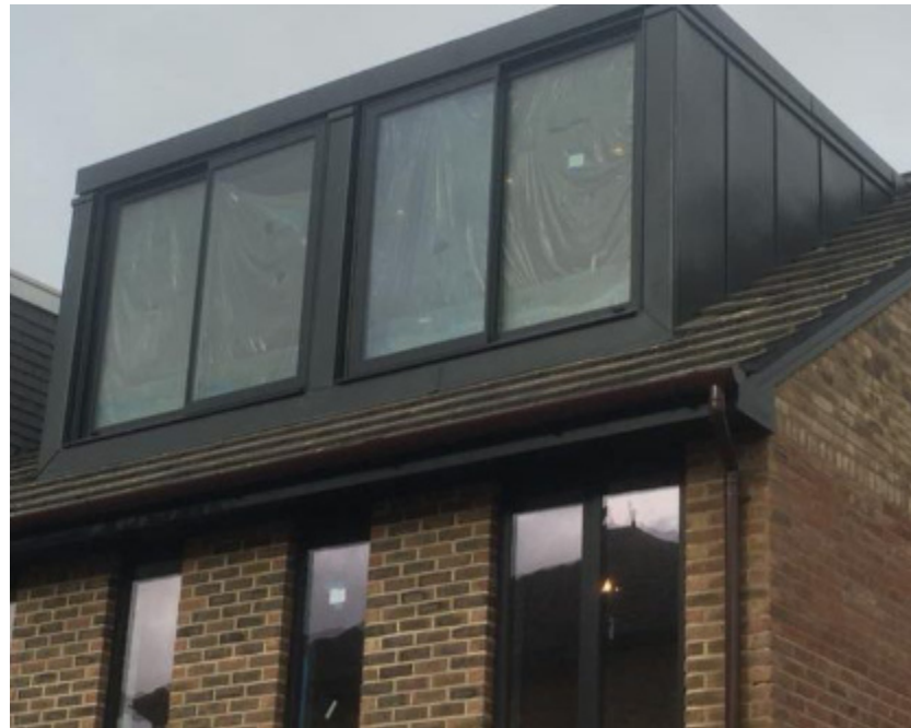
Standing seam dormer flat roof
