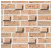
3 Dark snapper head brick detail
