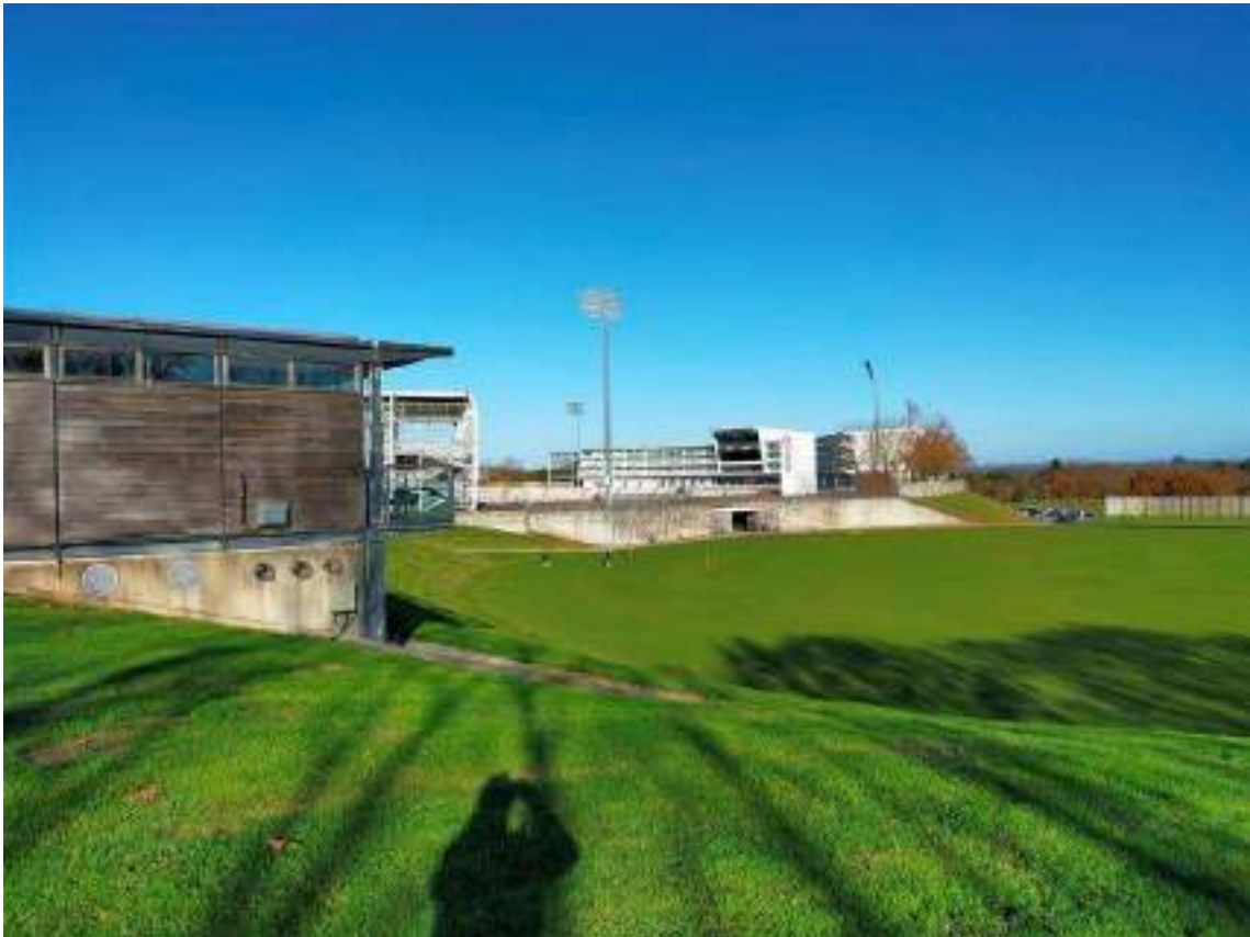
Photograph 40: General view North across training pitch, towards the stadium and proposed pavilion/budget hotel.
