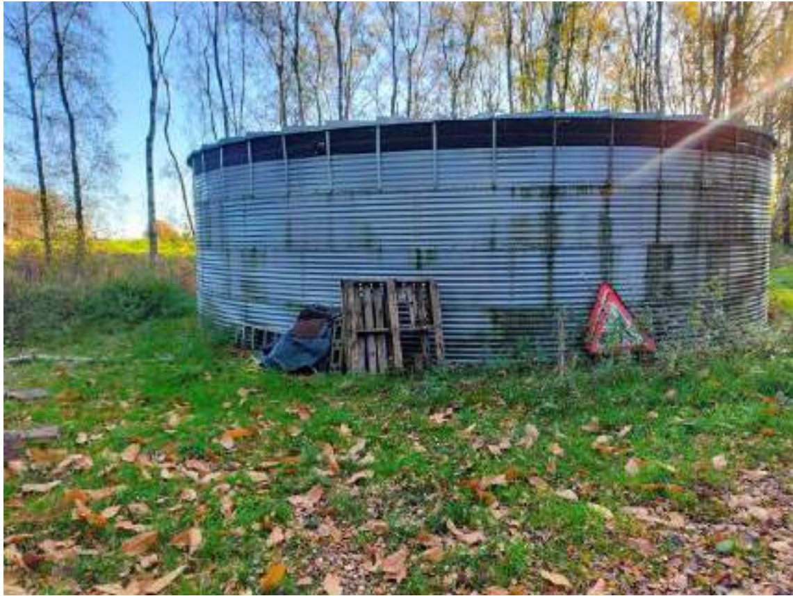
Photograph 15: General view East of storage tank behind Hickley Farm Cottages.
