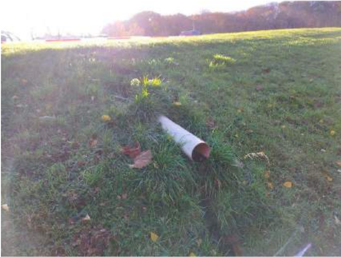
Photograph 29: General view South showing pipe draining car parking area into ditch along North Site boundary.
