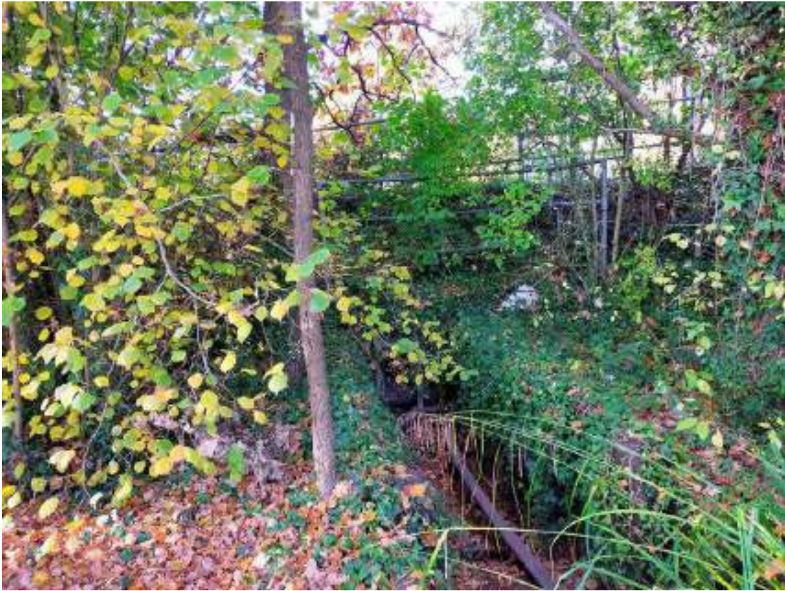
Photograph 23: General view West of drainage ditch leaving culverted section beneath Marshall Drive.
