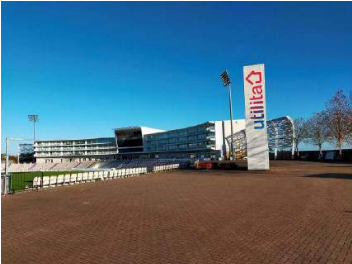
Photograph 2: General view North in the area proposed for the pavilion.
