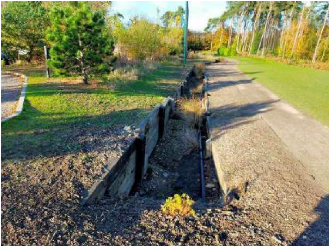
Photograph 22: General view West along the first fairway with drainage ditch lined with sleepers.
