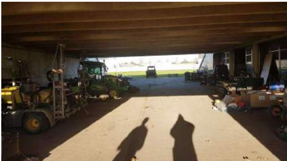
Photograph 4: General view ground floor access tunnel showing vehicle storage .
