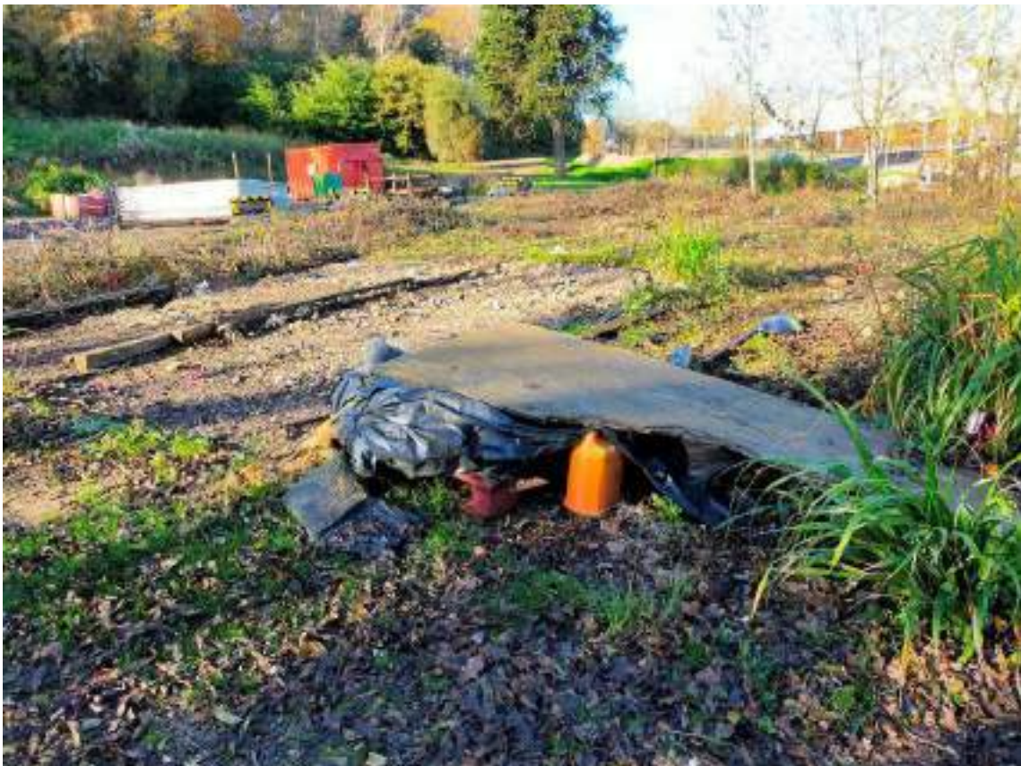
Photograph 36: General view North West across former site compound showing crushed demolition waste and general waste.
