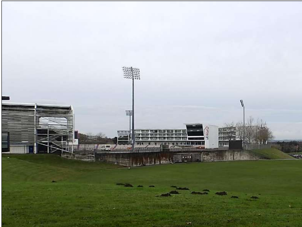
Figure 3.2 Character Areas 2 & 3 – Staff access, stands and turfed bank viewed from the south east
