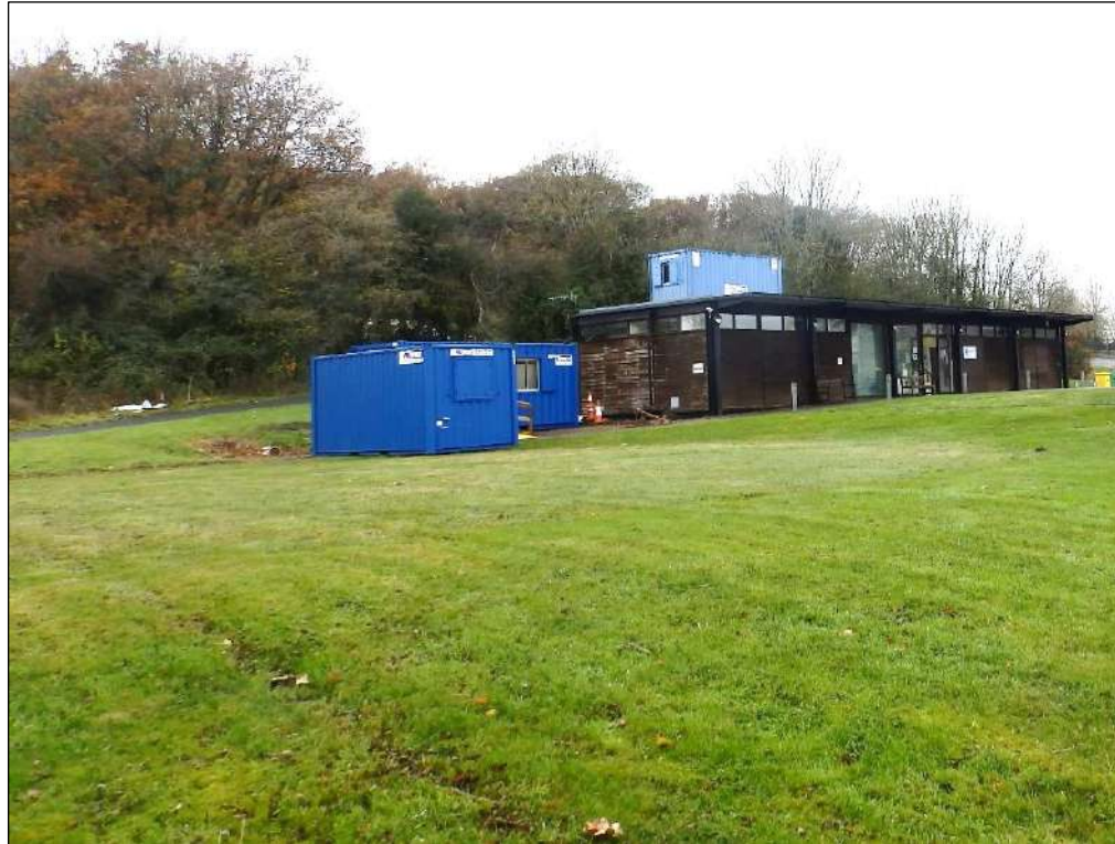
Figure 3.3 Character Area 4 – Hampshire Wellbeing Centre and temporary offices with woodland and earthworks compound beyond, viewed from south east
