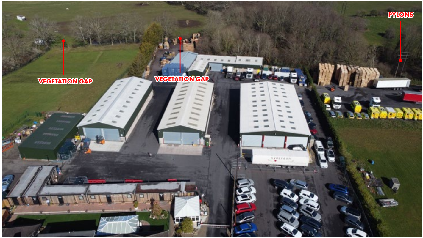
DRONE PHOTOGRAPH A VIEW TAKEN FROM THE CENTRE SECTION OF THE WIDER CCW SERVICES LOOKING NORTH SHOWING THE CONTEXTUAL ELEMENTS OF THE SITE COVERING THE EXISTING WAREHOUSES AND THE FIELD TO THE IMMEDIATE NORTH-WEST WITHIN THE WIDER CCW OWNERSHIP.
