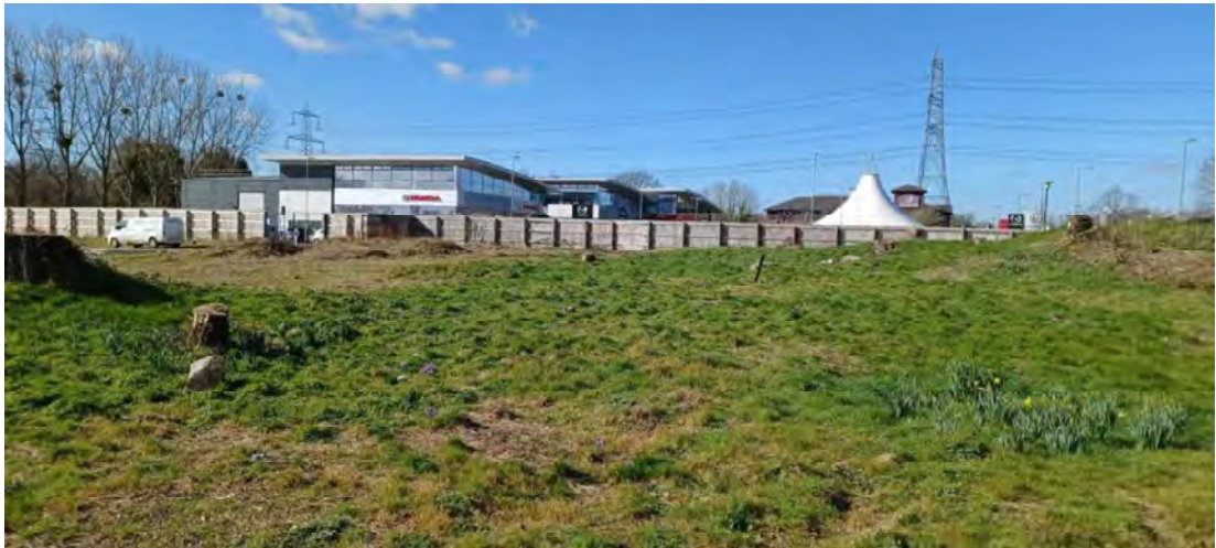
Northern half of hoarded part of the site, looking west
