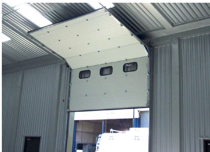
Example of sectional shutter - interior
