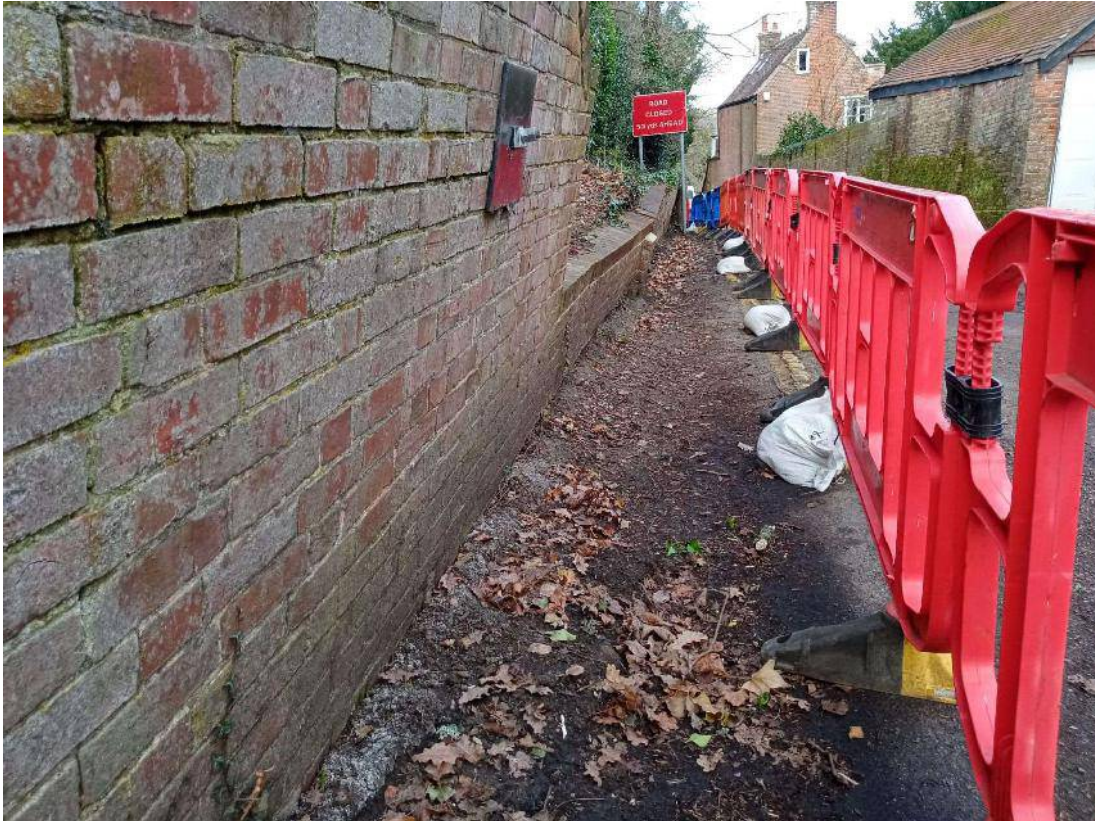
Photograph 4 – View along junction between wall Lengths A & B showing step in height
