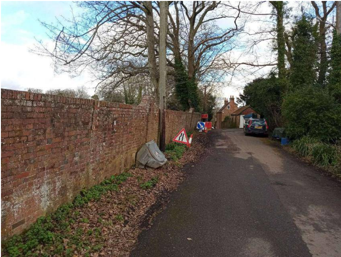
Photograph 1 – General view of Southern end of wall
