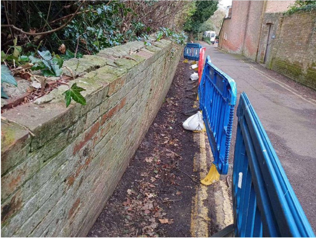
Photograph 7 – View along wall Length C
