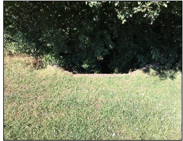
Figure 13 Image showing the end of the culvert and beginning of the ditch
