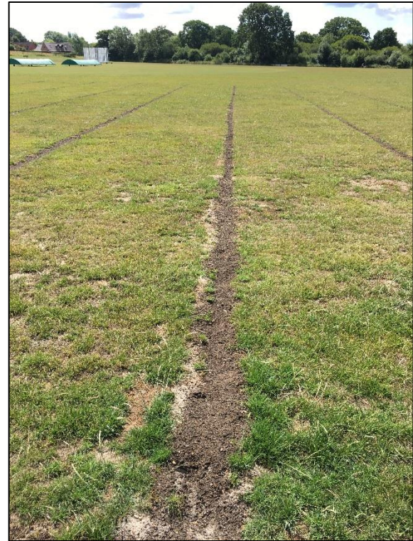
Figure 11 Sand slits entering the collector drain
