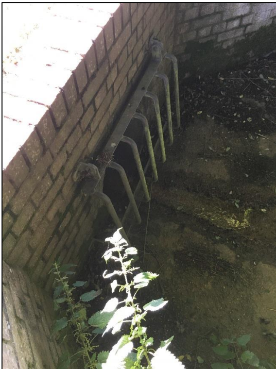
Figure 14 Close up of the culvert
