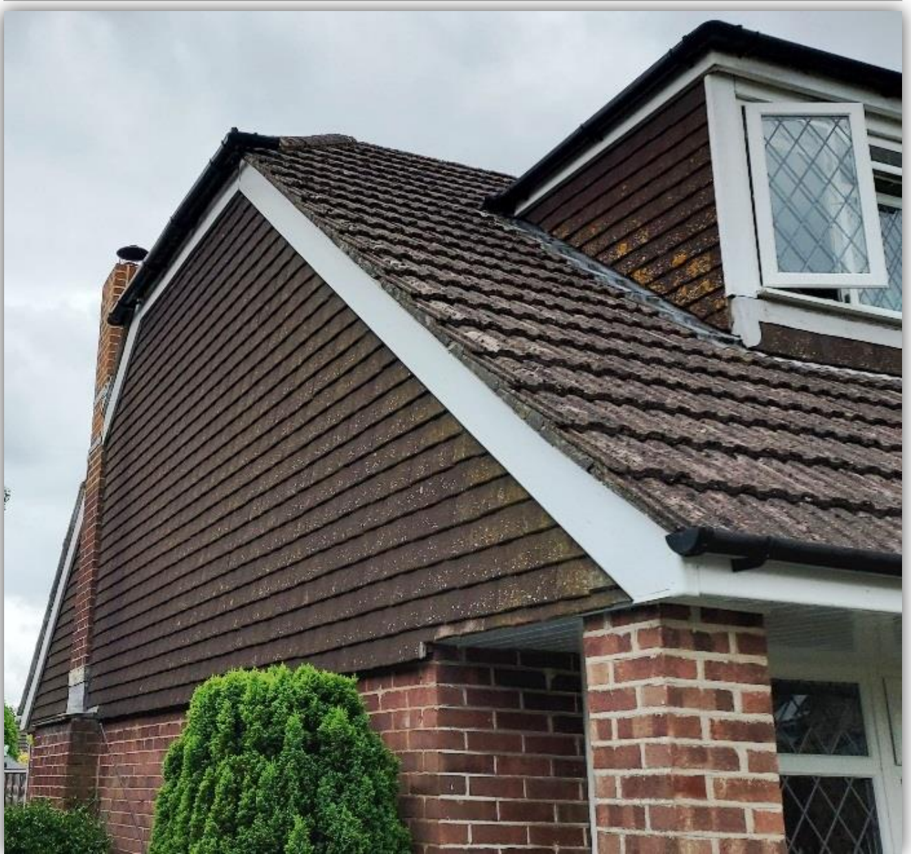
Side (east) elevation and hanging tiles.
