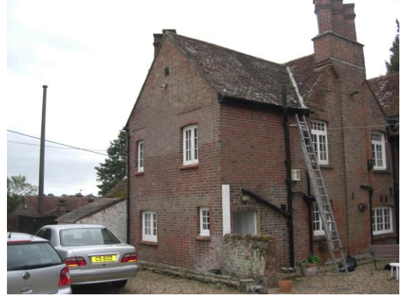
North wing and adjacent parking area
