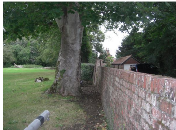
Mature tree abutting the wall
