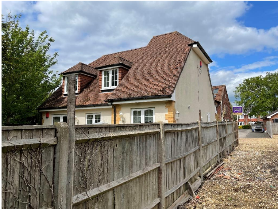
Rear Elevation of 57 Pound Lane
