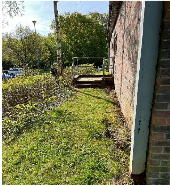
The existing grass fire escape path
