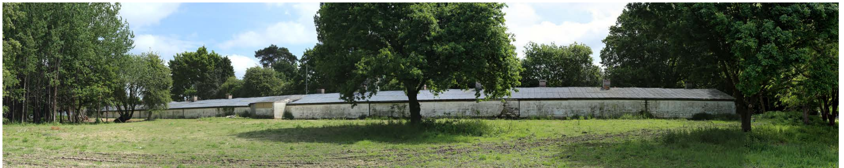
Site View B - looking east
