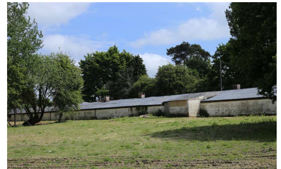
Existing Cockpit Farm building
