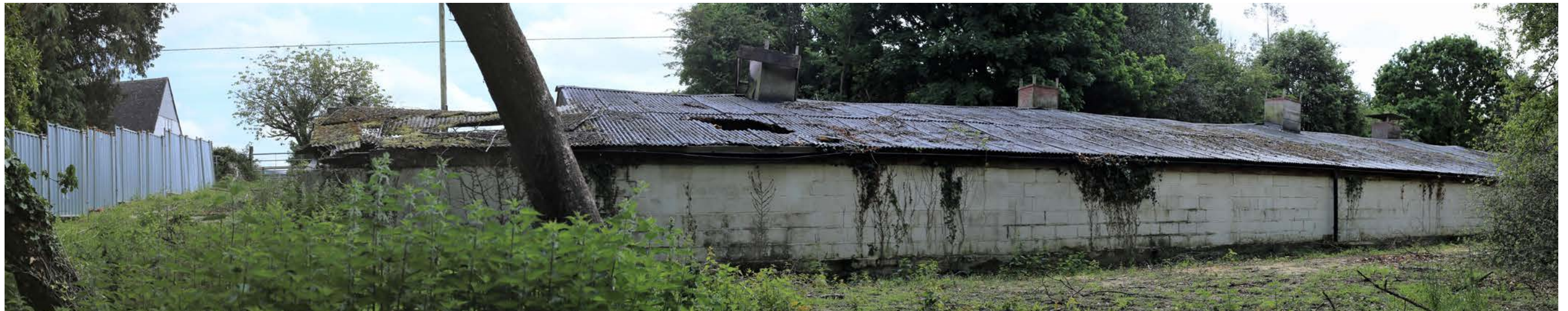
Site View A - North west corner of the site
