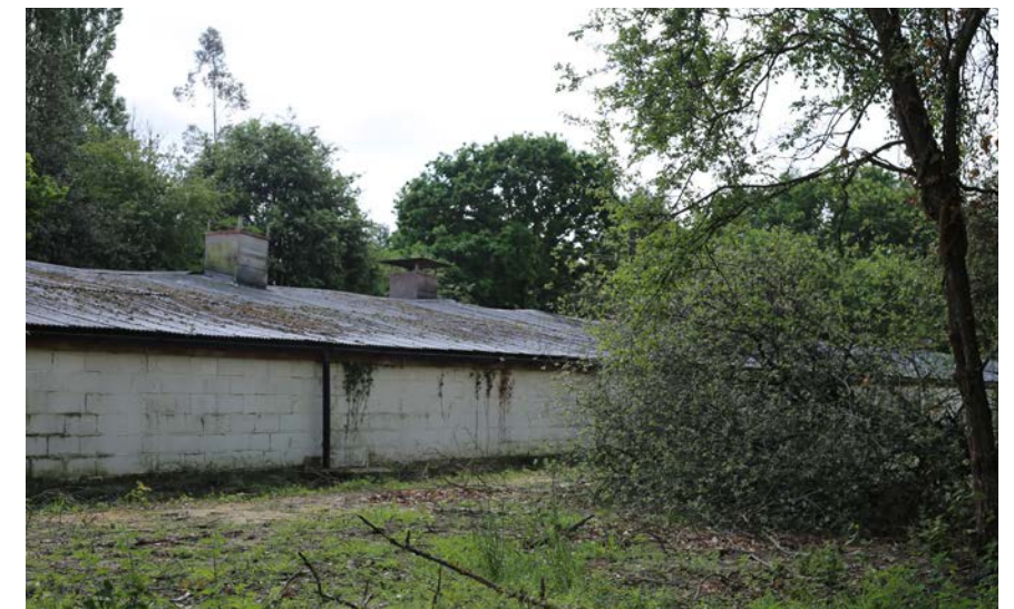
The site is in poor condition
