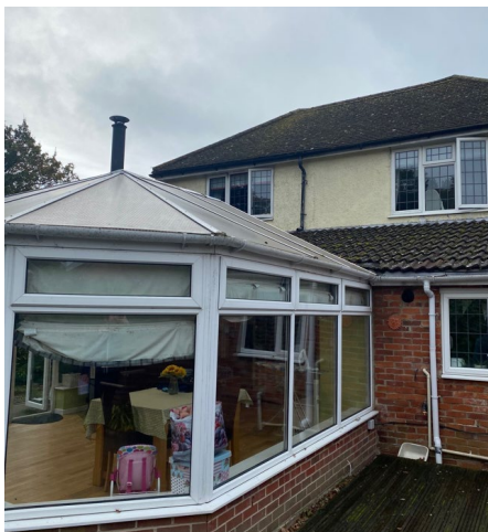
View rear left of building
