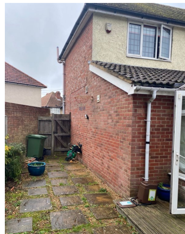
View of rear right of building
