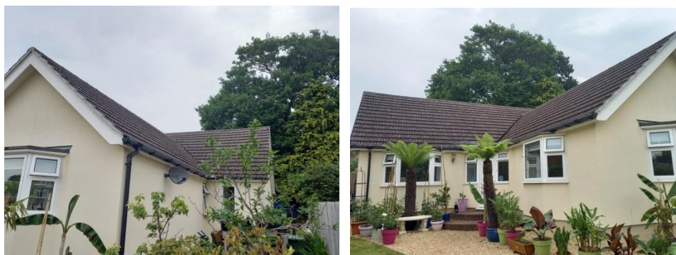
Front elevations, showing good condition of bungalow walls/roof
