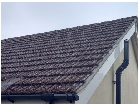
Tightly-fitting roof tiles & sealed verge /soffits throughout
