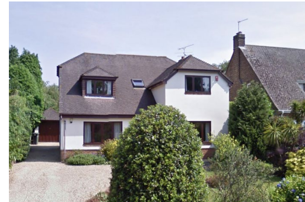
Fig.8 – 12 Grosvenor Road – rendered walls; cropped hip and swept roof
