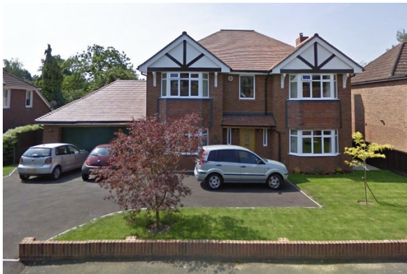
Fig.9 – 3 Grosvenor Road – bay windows with faux framing to rendered gable infill; symmetrical frontage
