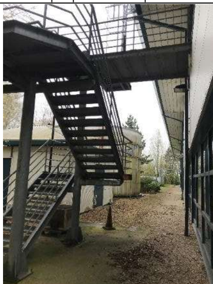
09 External stair to north side
