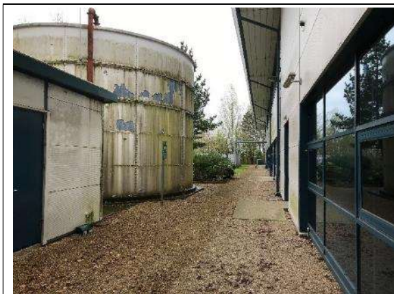
07 Foul water pump station and sprinkler tank
