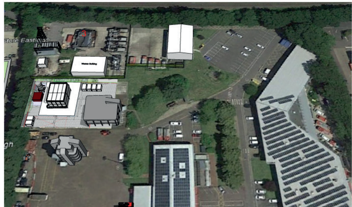
Site Works - Overview
