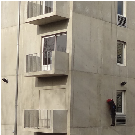
1. External Finish Pre-Cast Concrete Slab
