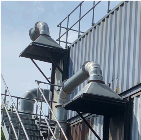
4. Grille / Vent Flues Steel to Withstand Heat
