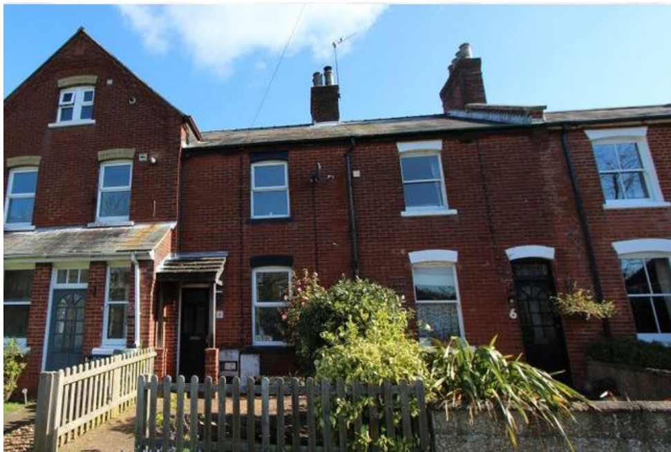
No.4 Station Road, Netley Abbey, SO31 5DT
