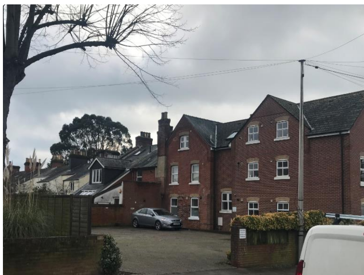
The rear of No.4 Station Road, view from Station Road
