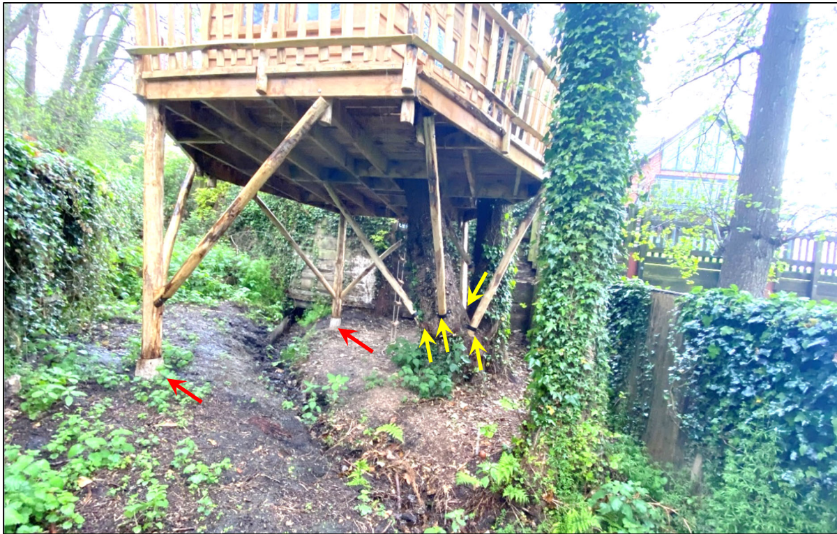
Figure 2: View of the tree house from beneath looking towards the house and the retaining structure at the end of the garden, with the small concrete piles shown by the red arrows. There are further supports fixed to the tree trunk with brackets shown by the yellow arrows.
