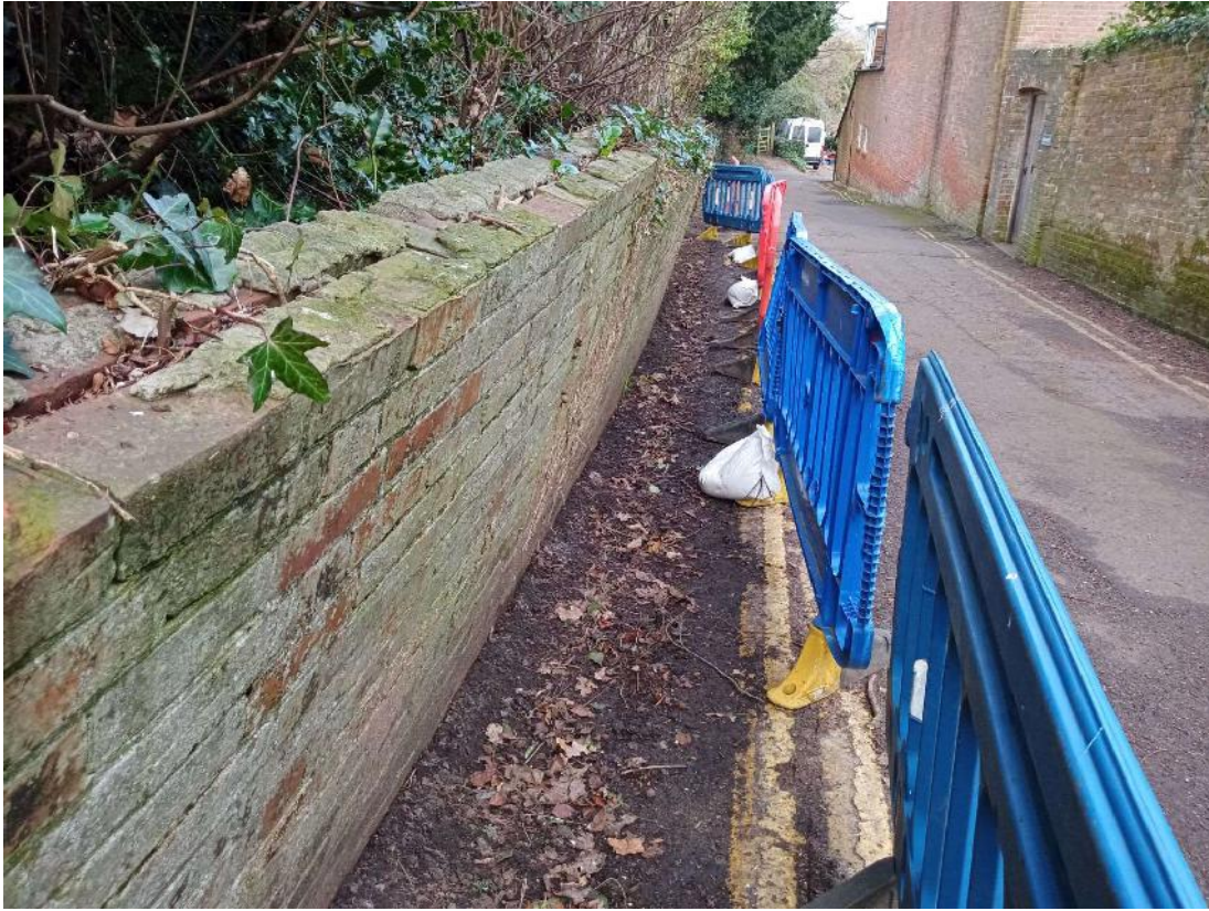
Photograph 7 – View along wall Length C
