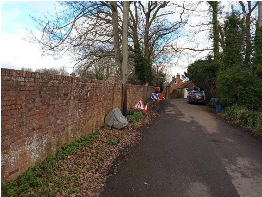
Photograph 1 – General view of Southern end of wall
