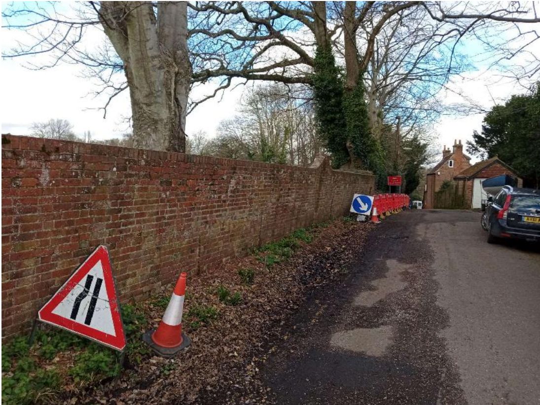
Photograph 2 – General view of wall Length A
