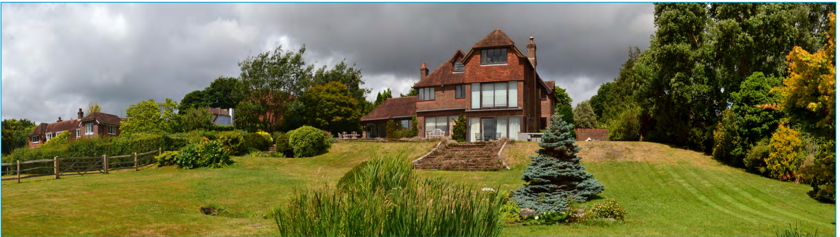
View B from the centre of the site looking north-west to the southern facade of existing dwelling.
