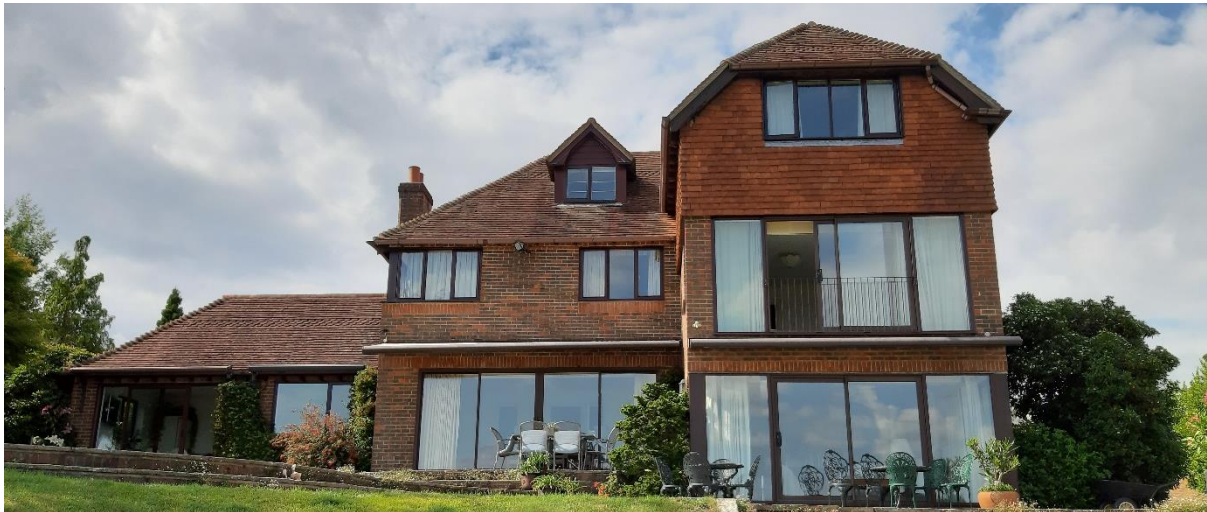
Photo 1: South-eastern elevation of the house showing hanging tiles at first and second floor level
