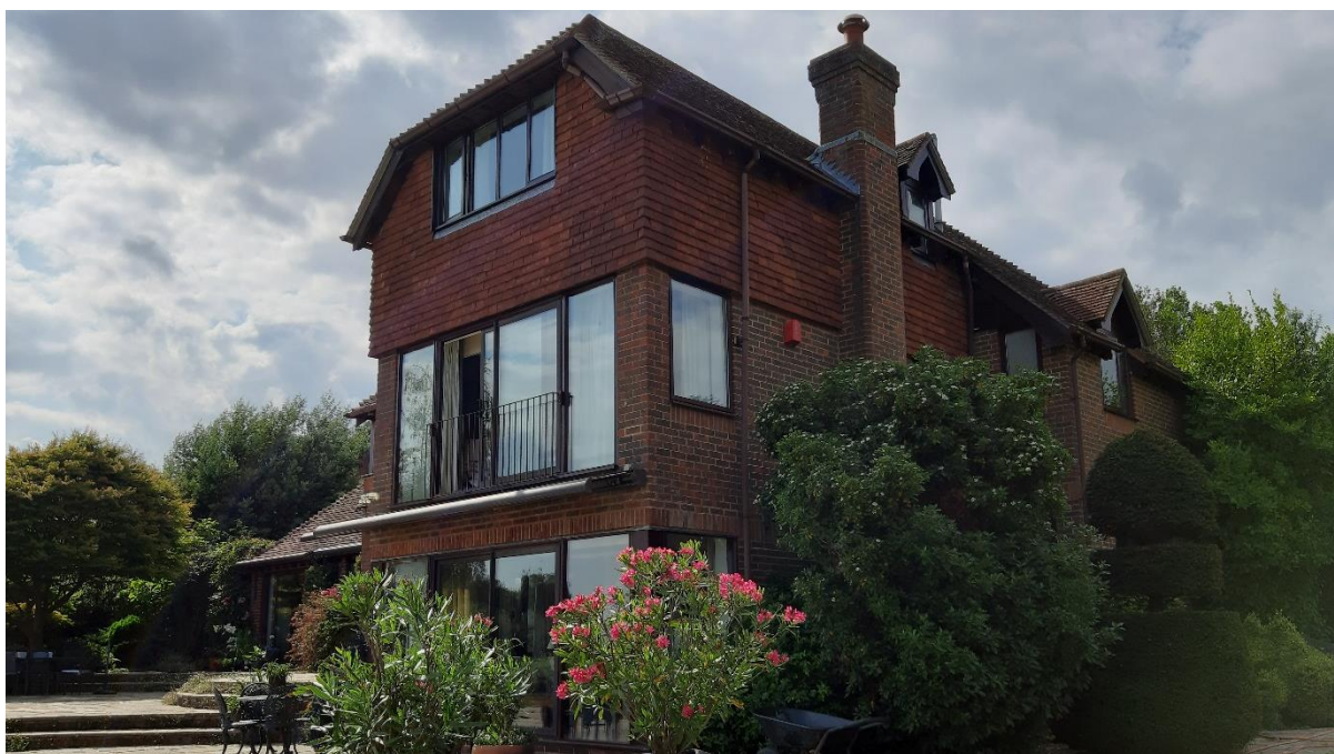
Photo 2: The north-east and north-west elevation with hanging tiles on second floor
