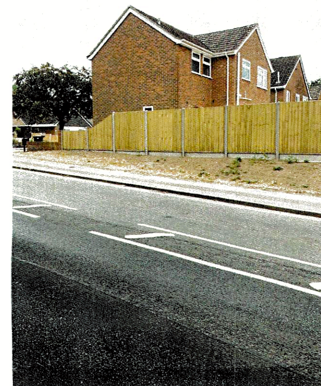
view of fence from mortimers lane
