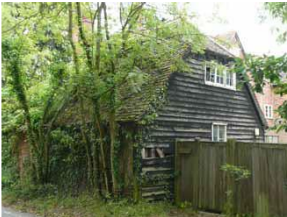
Existing Barn and Access at Maidenstone Heath
