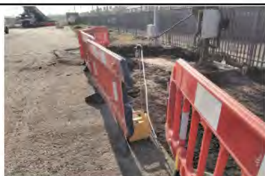
West boundary line location A AB37 25.03.22 09.20
