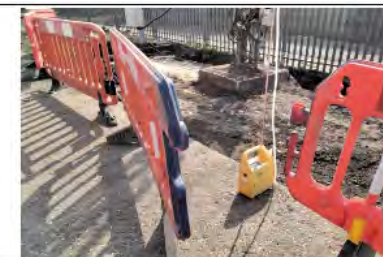
West boundary line location D AB35 25.03.22 12.38
