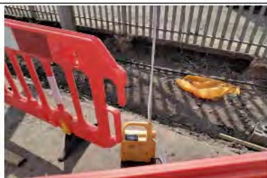
West boundary line location A AB37 25.03.22 12.35
