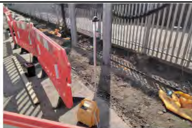
West boundary line location A AB37 25.03.22 11.27
