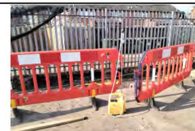
West boundary line location D AB35 25.03.22 09.25
