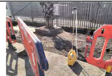
West boundary line location D AB35 25.03.22 11.30
