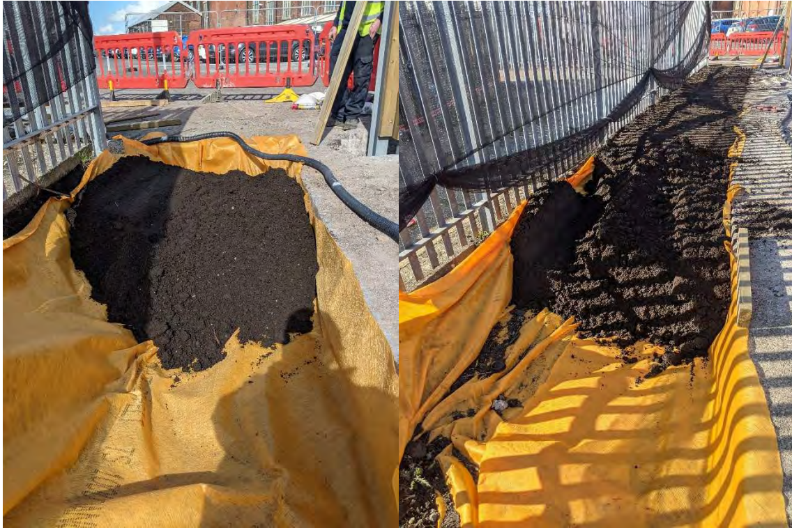
Photographs 9a & 9b - Application of clean cover system on top of geotextile membrane.
