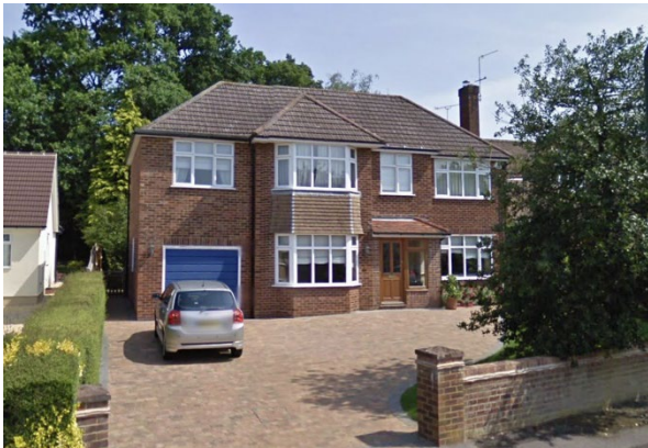
Fig.6 – 4 Grosvenor Road – 2 storey hipped bay window and integral garage
