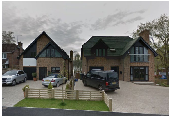
Fig.10 – 125-127 Kingsway – contemporary style with glazed gables and Juliet balconies
