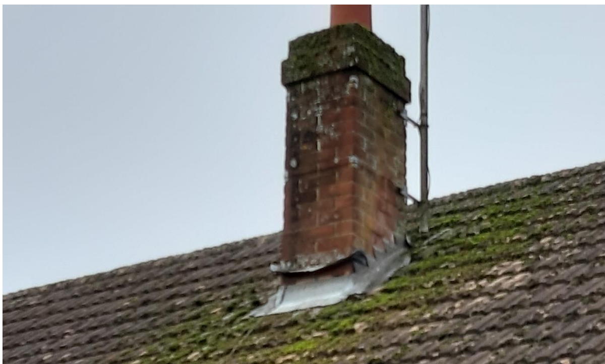
Photo 3: access around the chimney in 2020
